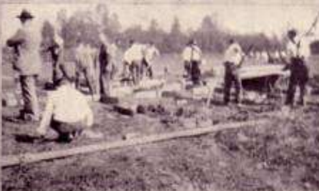
Grandstand in the Making
